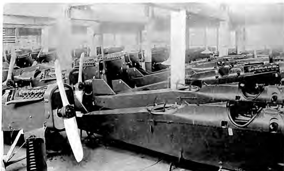
Group of De Havilland-4 fuselages ready for final assembly of wings, center sections, and tail surfaces
