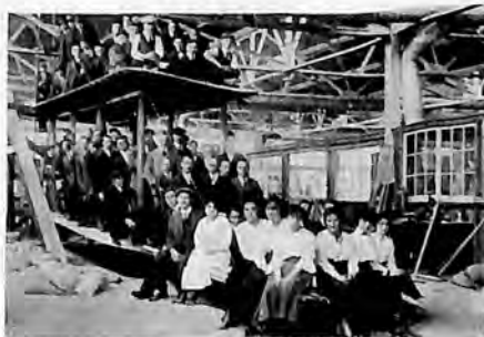
Live Load Test H-12-A Panels
