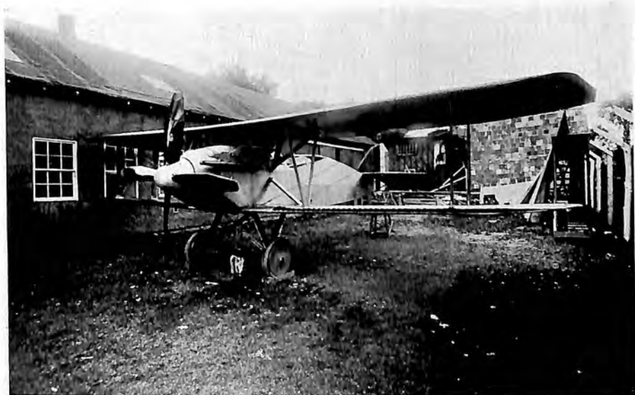
MB-2 Fighter, Two-Place, with 450 Geared Liberty Engine
