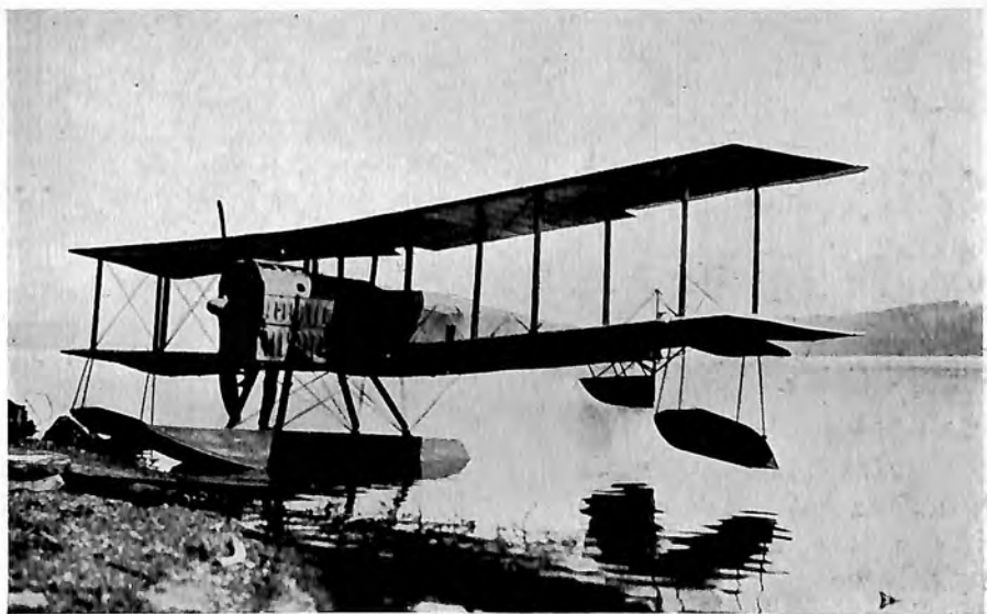
D-2 Hydro-aeroplane, with Thomas 135 H. P. Engine
