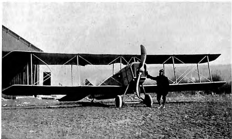
Model D-2 Two-Place Tractor with 135 H. P. Thomas Engine
