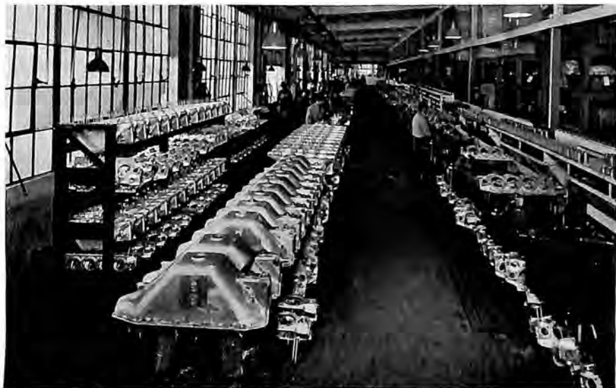
Looking Down one of the sides of the Assembly Floor from the point where the Finished Crankcase starts along the line
