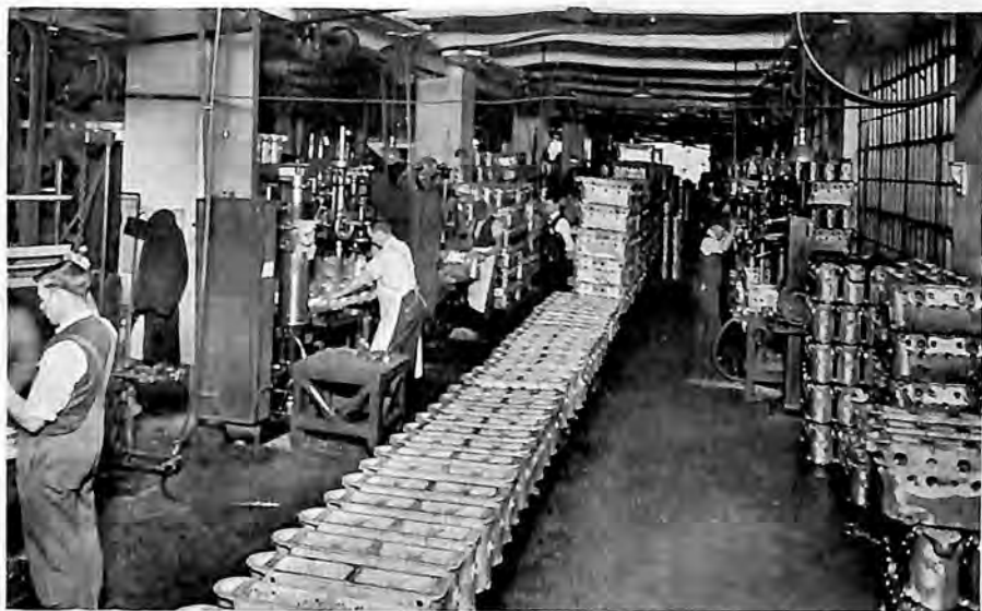
Machining line for the Aluminum Water-Jacket Casting in the Wright-Martin Foundry
