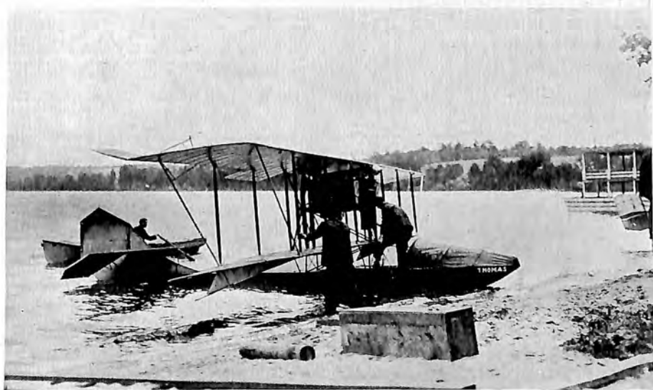
The Original Thomas Flying Boat with 65 H. P. engine
