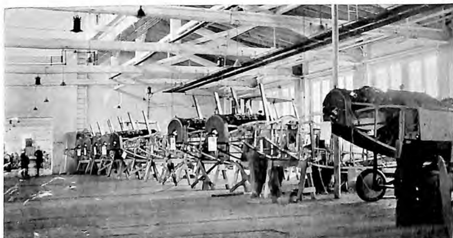
Fuselages ready for covering in the Springfield factory
